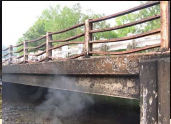
Gasoline that spilled from the tanker-truck accident on the bridge over the Norwalk River near Ridgefield, Conn., caused spalling on the precast concrete but left it in "reasonably good shape," engineers reported.
